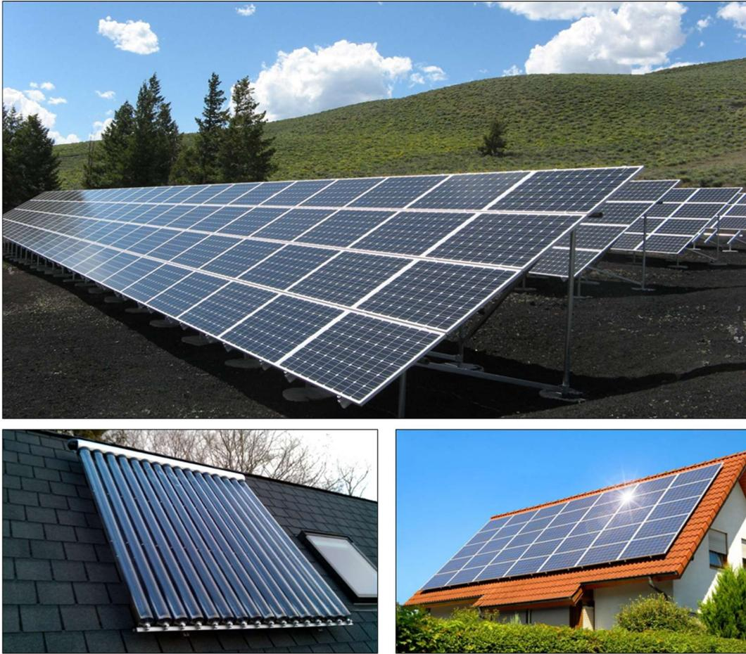
**Figure 3-1:** Examples of solar energy installations: ground mounted PV installation (top); rooftop mounted solar thermal (bottom left); rooftop mounted PV (bottom right).
